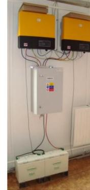
Fig. 3. Connecting the Hopecke batteries to the SunnyIsland converters.
